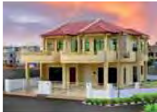
Double storey show house
