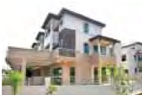
Three Storey Terrace House
